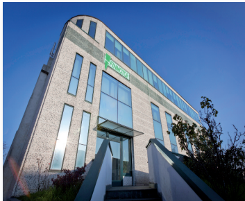
Enerdoor/Finmotor headquarters Milan, Italy
